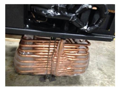
Smaller Ice Bank for CO<sub>2</sub> Refrigerated Dispenser at a lower ambient condition
