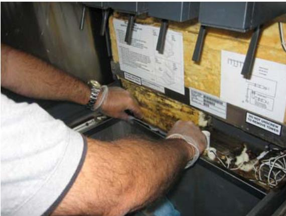
24. Rotate barrier into position, if necessary bending the left side out to slip it into place.
