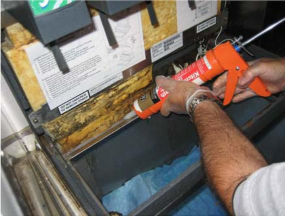
22. Silicone the lower barrier per the image below.
