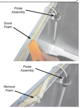
7. Run the probe assembly wire along the channel cleared of foam in the previous step.
