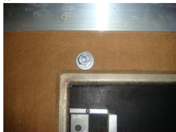
4. Apply a bead of silicone around the mating surfaces of the dispenser to counter and clean any excess to present a neat appearance
