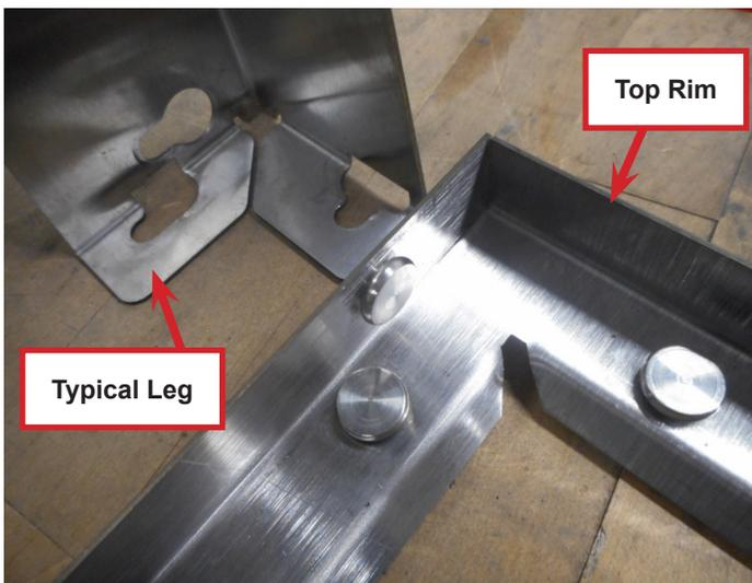
2. Align keyhole slot of leg with the rim button against inside edge of the top rim.
